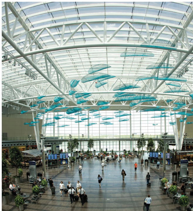
Midfield Terminal, as pictured in an Airport Authority financial report: Radiant floor cooling saves energy in a 60-foot-high space.
